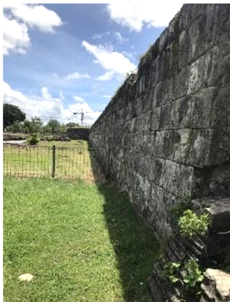
Figure 4. One corner of the remaining Surosowan Palace fort showing the walls built of coralstone (photograph by Rismawidiawati, 2022).
