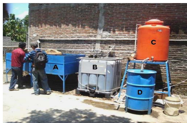
Figure 1. Wastewater Treatment Reactors, i.e. ABR (A), RBC (B), Collecting Tank (C), and Filter (D)
