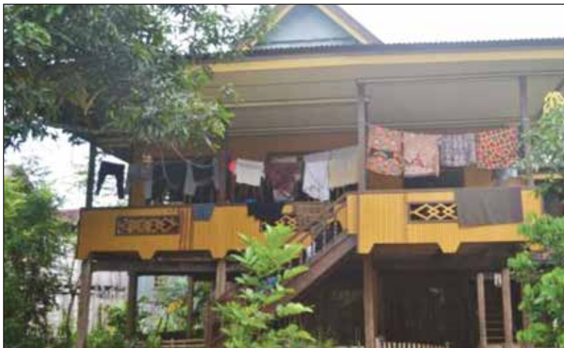
Picture 7a. The front section of HJ. Nemma's house (photograph by the authors, 2014).
