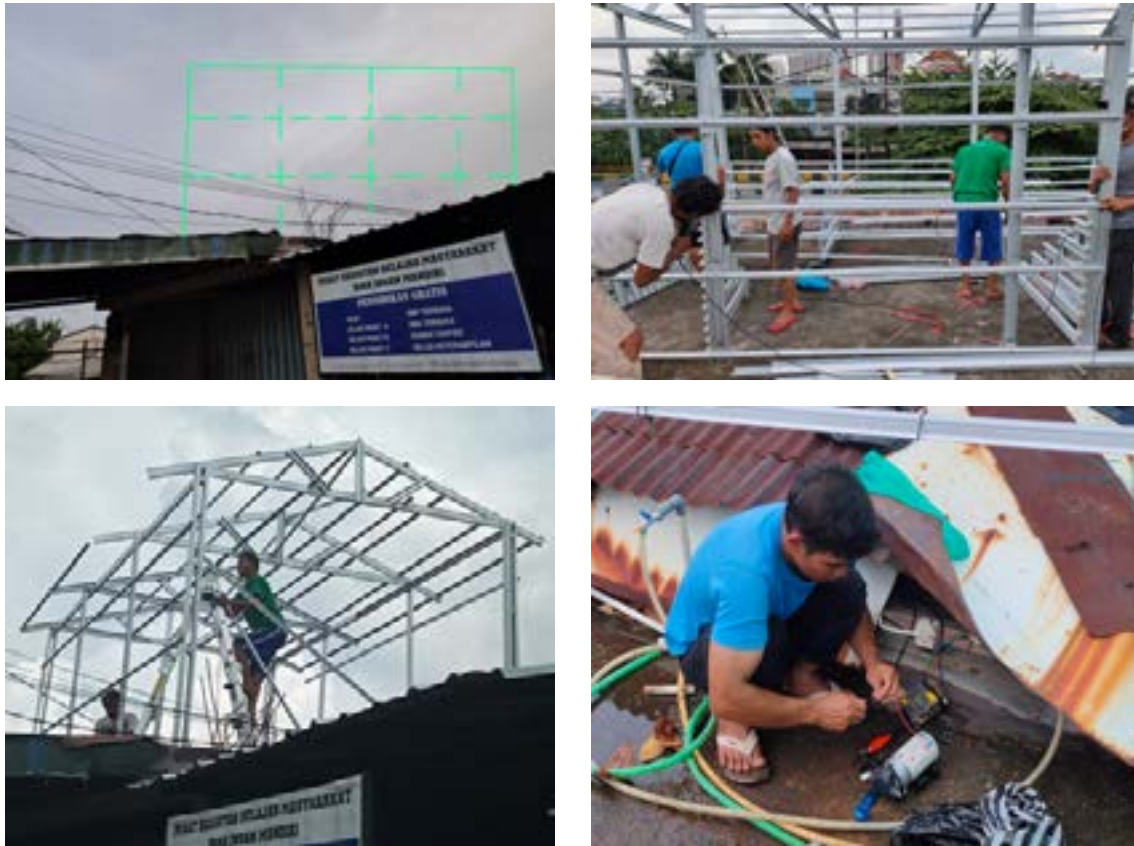
Figure 3. The construction of greenhouse and installation of automatic watering system.
