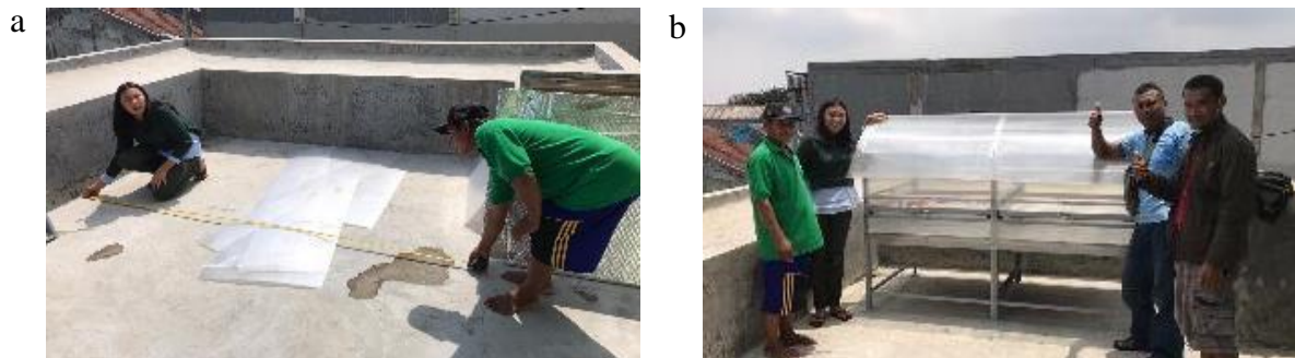
Figure 2. (a): Measurement of drying area; utilizing the roof of one of the farmers' houses to get as much sun as possible. (b) Finished product of modified solar dryer
