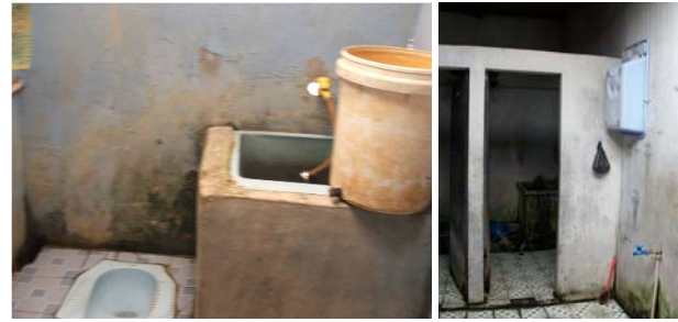
Figure 8. Sanitary Facilities in Some Houses
