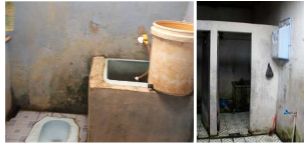
Figure 8. Sanitary Facilities in Some Houses
