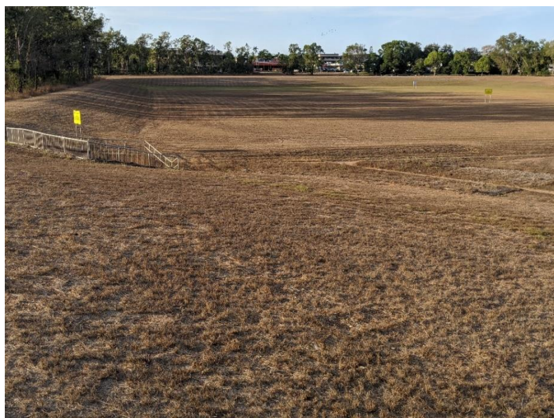
Figure 7. Rapid Creek stormwater retention basin
