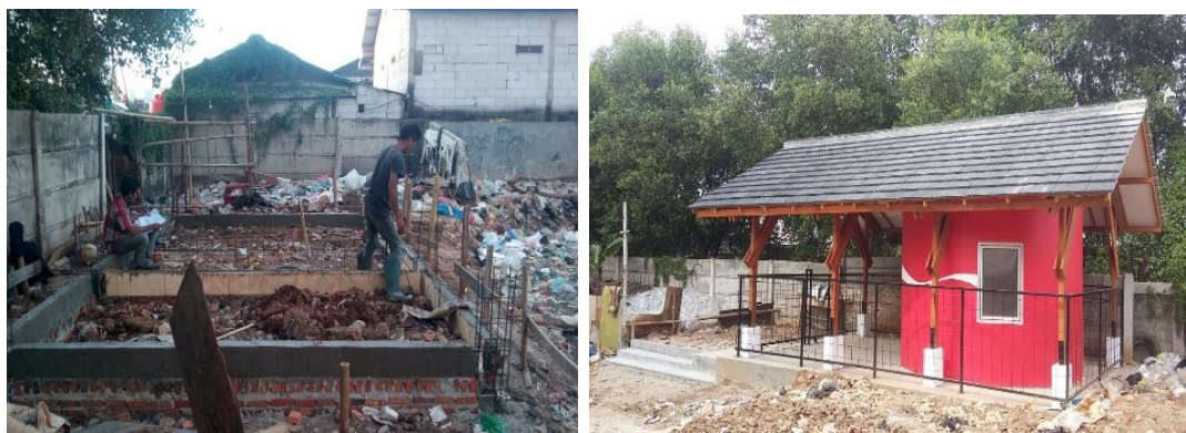
Fig. 4 Waste bank before and after construction
