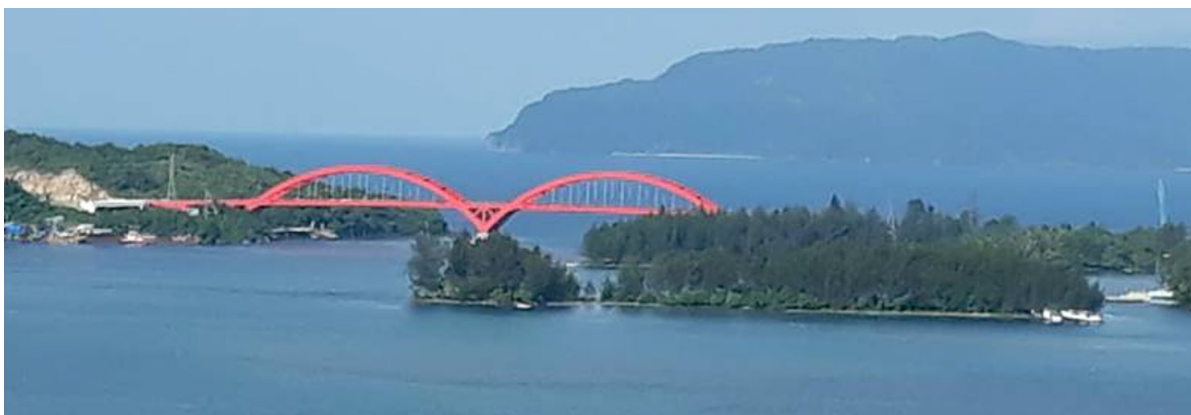
Figure 2. Holtekamp Bridge Source: Processed by the author (2018)
